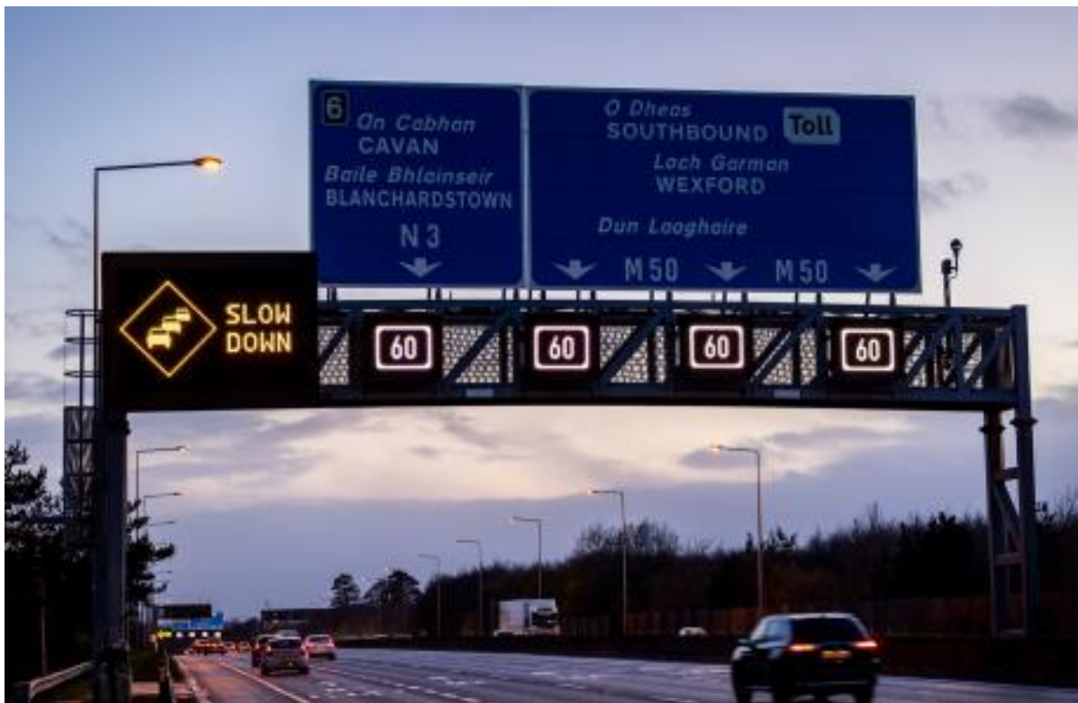
M50 Variable Speed Limit
